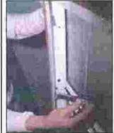
Install new balance assembly by reversing the removal procedure. Insert terminal clip in square hole located in frame jamb. Secure the lop guide under the take-out clip. Repeat on other side of window.
